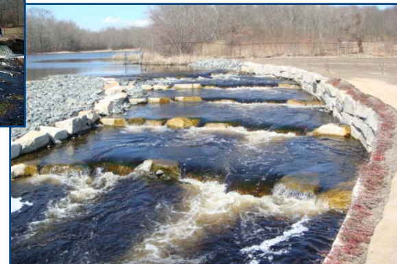
Dam Removal with Step-Pool Fishway
