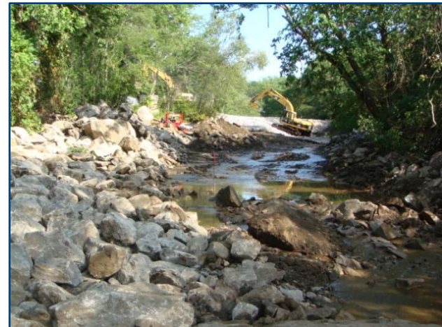
Dam Removal with Backwater Weir Installation
